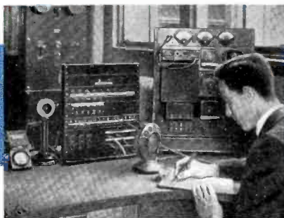
1922. One of the earliest audio systems, shown here at WWJ, Detroit, used a Western Electric 8-type amplifier, with keys, jacks and plugs provided for line selection and output switching.
